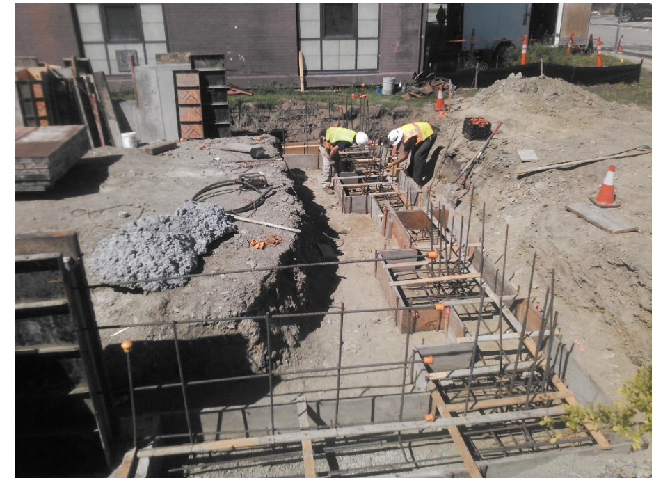
Load Bearing Concrete Footings
